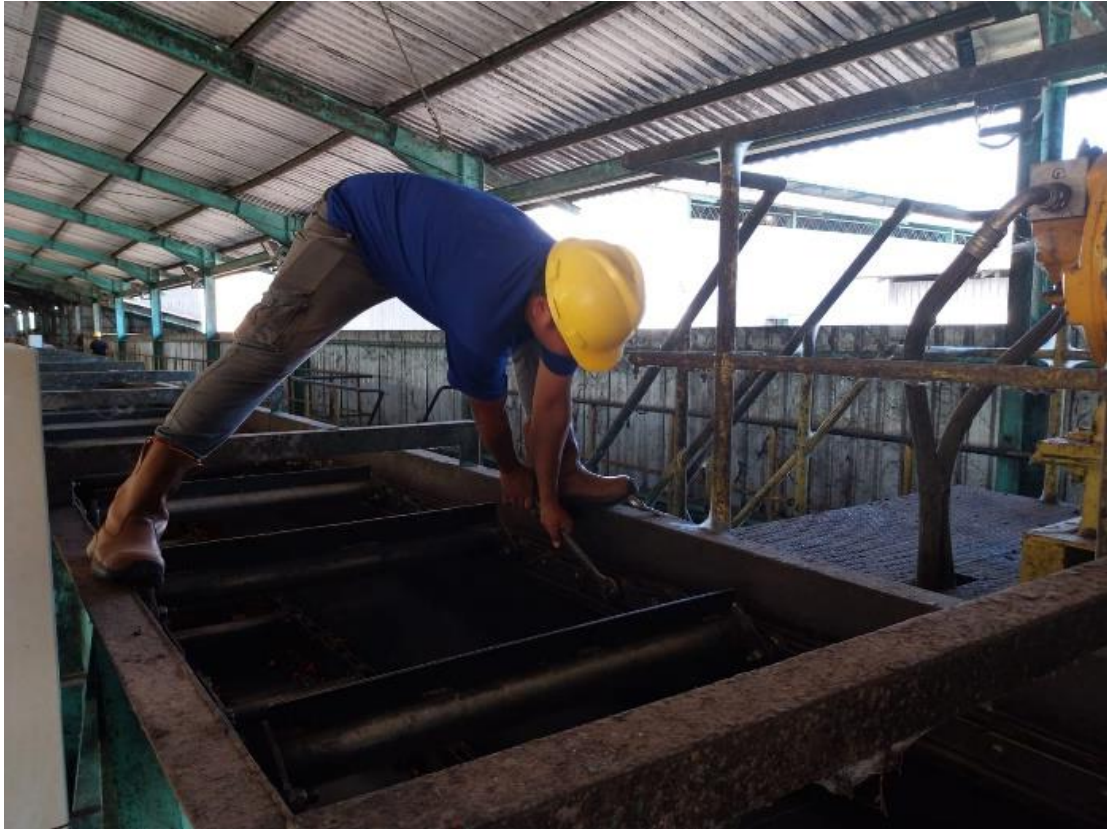
Gambar 1. Mekanik Preventive Baut Chain Screper Conveyor No 2
